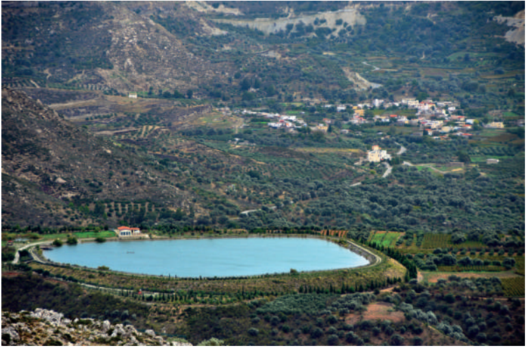
Gergeri, 'Digeni' reservoir
